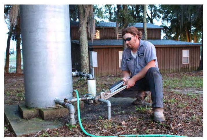
I am tightening up the 1" union after installing a new 1" brass ball valve to this water system that feeds an agricultural shop. The union allows for quick disconnect to save some time if the tank should ever be replaced while the valve in the photo will serve as a cutoff to individual lines which will allow us to fix lines without cutting off all water supply.
