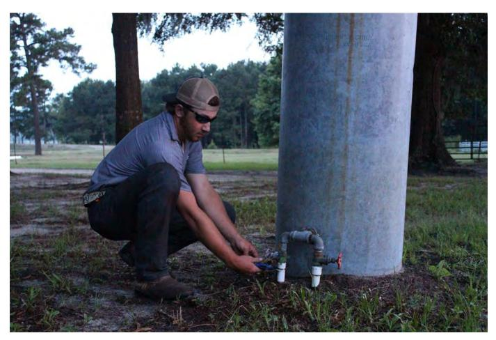
At this farm, I am fixing a 1" water line that froze and burst due to the lack of insulation. This line runs water to multiple cow troughs. It is critical to do this quickly and correctly to ensure that the livestock have water as soon as possible. After the line is coupled and glued back together you should ease the water on slowly to assure that there will be no more leaks in the water line.
