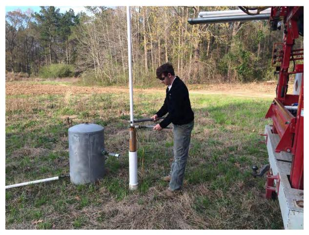
I am installing a 1 horsepower submersible pump as a residential application. Once we determine what the well will be used for and depth of aquifer, then I can decide and plan what equipment will be needed to supply the necessary water. This is will also include pipe size/length and tank capacity.
