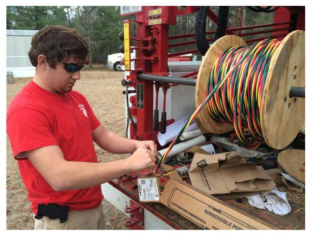
I am wiring the 12-3 pump cable to run with the pipe to carry the current from the control box to the 1 horsepower pump. By using the proper tools, such as wire crimpers I can guarantee that the bonds between the cables will be water resistant. This connection shall be made with connectors and then covered with a plastic that will ensure the seal that is needed for proper performance.
