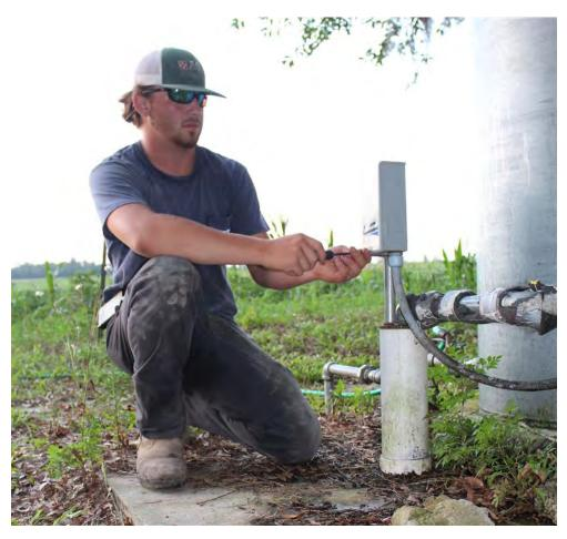
Having an understanding of electrical wiring has been essential to my job. In this photo, I am wiring a pump to the new control box outside of this farm shop so the pump will have power to run and supply water to the facility. This box is essential to the installation due to its ability to prevent early failure of the pump motor below.
