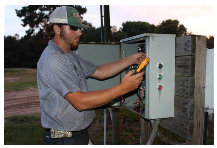
I am using the voltage meter to troubleshoot this service call. Understanding the entire well layout, as well as how the well works from the ground up, is important in problem solving because certain parts can fail. Checking the voltage is usually where I start. Even if the voltage is correct before the motor is running, you need to start the motor to assure there is no voltage drop while it is running.
